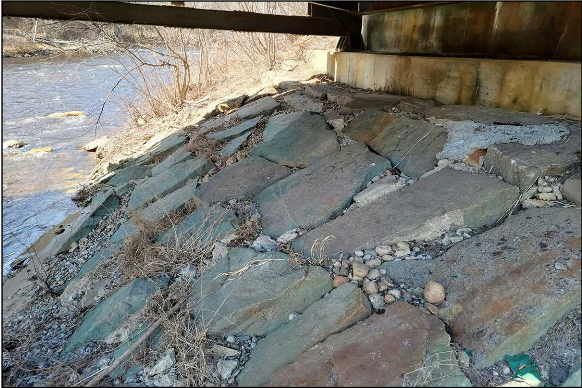
PLATE 2: Stones Brought in to Construct Eastern Abutment, View East
