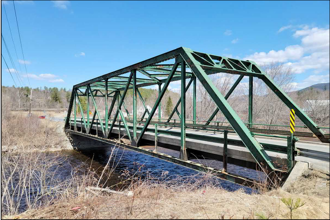
PLATE 1: Bloomfield Bridge No. 9, Facing Northeast
