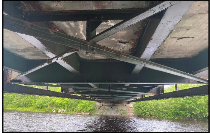
Figure 1-6: Typical Floor System Condition
