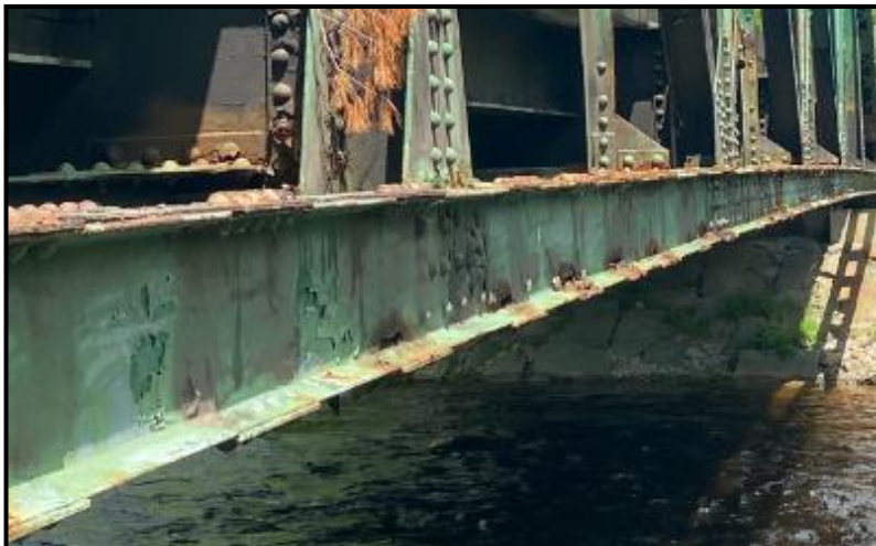
Figure 1-5: Typical Deterioration in the Bottom Chord
