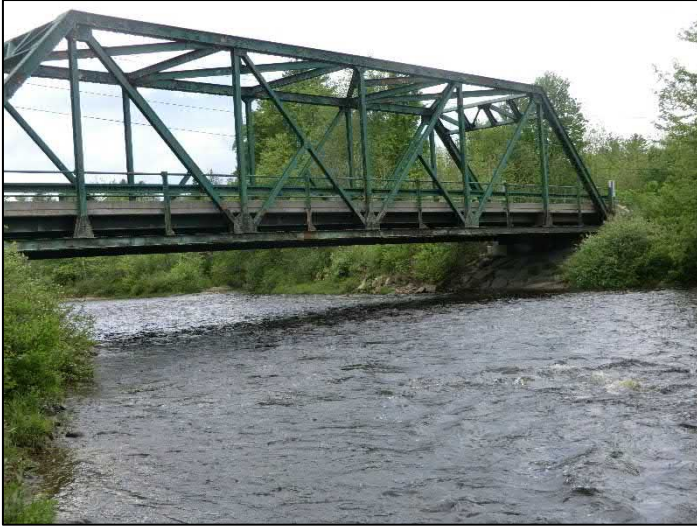
Figure 1. Route 102 Bridge (looking downstream)
