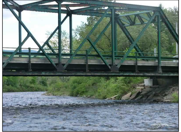
Figure 2. Route 102 Bridge (looking downstream)
