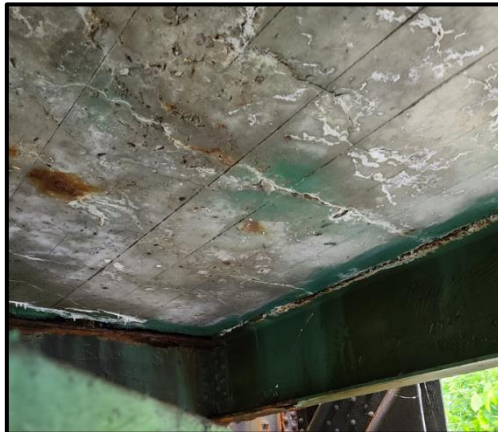
Figure 1-12: Typical Underside of Deck
