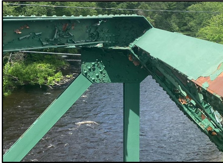
Figure 1-2: Typical Repair of End Post (Top Left)
