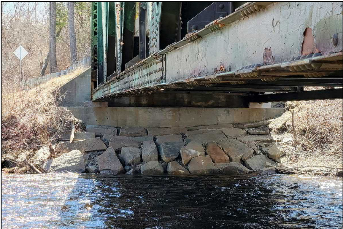
PLATE 3: Stone Brought in to Construct Western Abutment, View West
