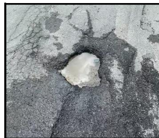
Figure 1-15: Small Pothole in Travel Way (Below)
