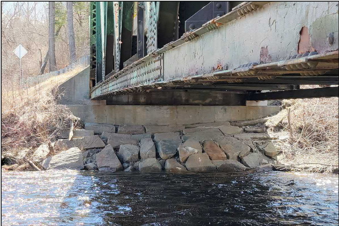
PLATE 3: Bloomfield Bridge No. 9, Facing South
