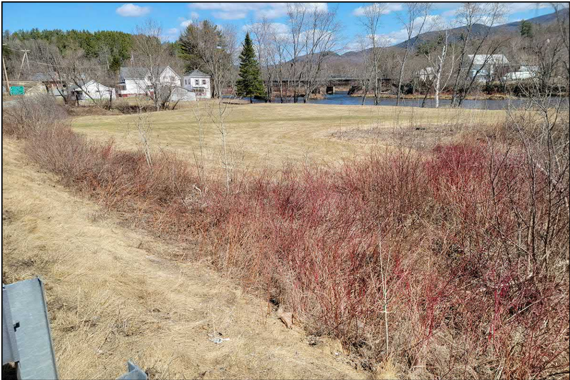
PLATE 1: East Portion of APE Showing Buildup of Roadway Leading to Bridge, View East
