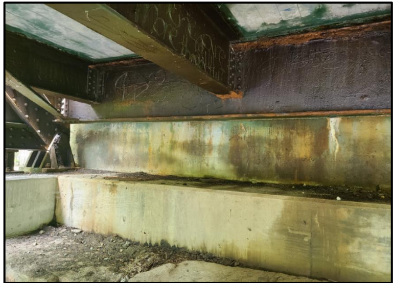
Figure 1-17: North Abutment and End Framing in Good Condition
