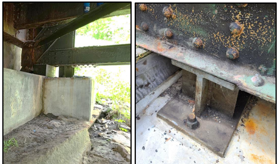
Figure 1-9: South Abutment and Bolsters
