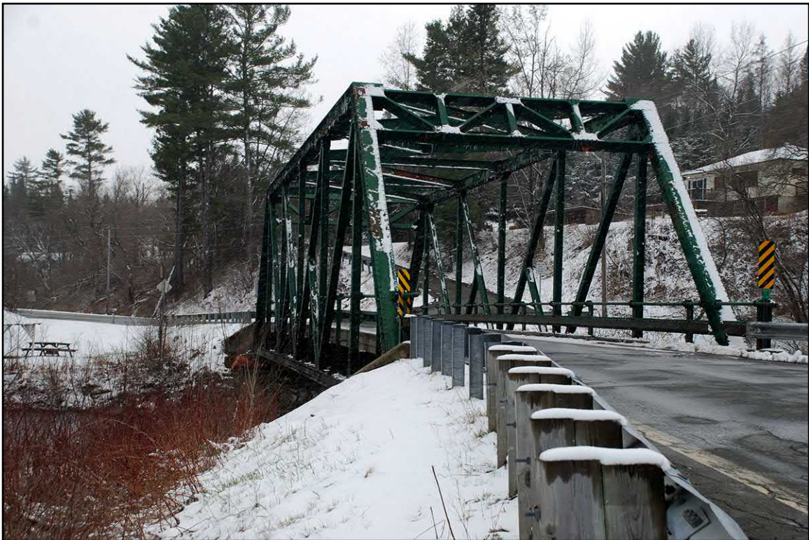
PLATE 2: Bloomfield Bridge No. 9, Facing Southwest
